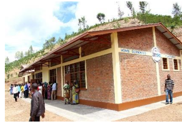
Home economics classroom exterior
